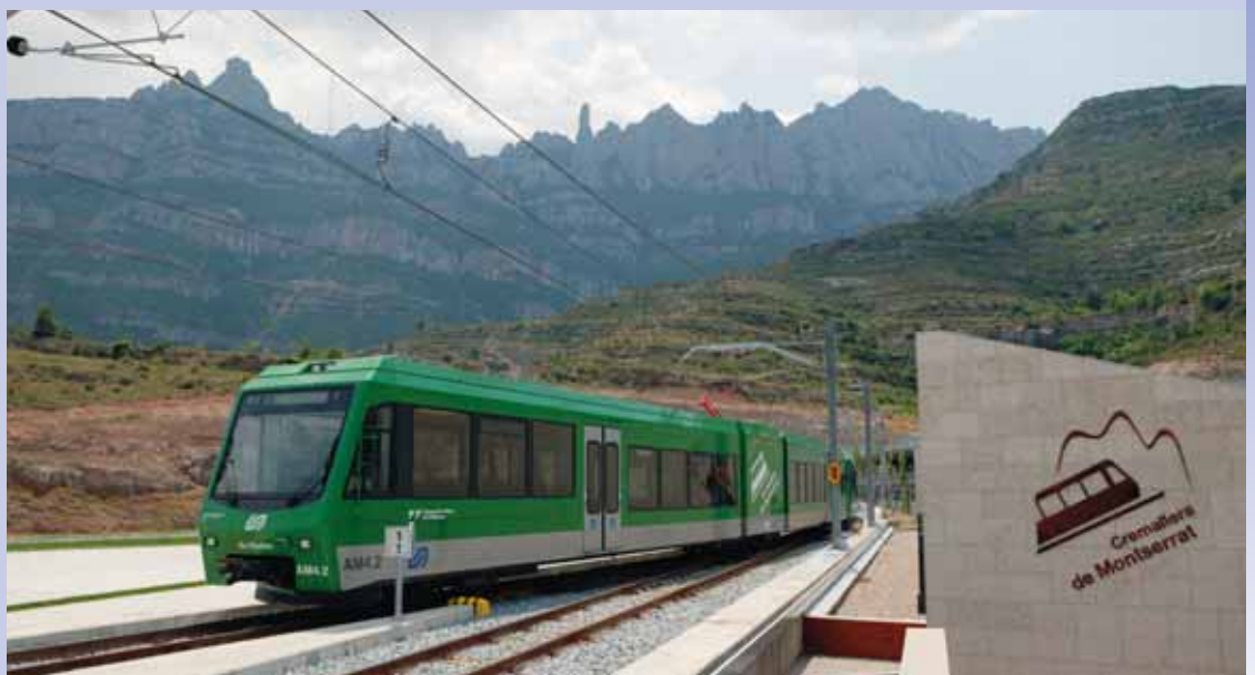
Rackrail at Montserrat, Spain
